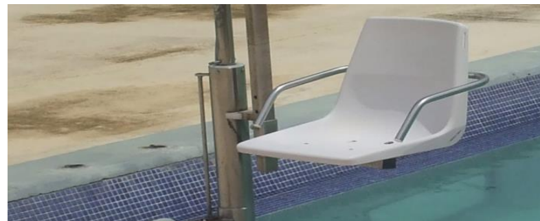
INSTALLATION OF HYDRAULIC POOL LIFT CHAIR DIEGO MARTIN SWIMMING POOL
